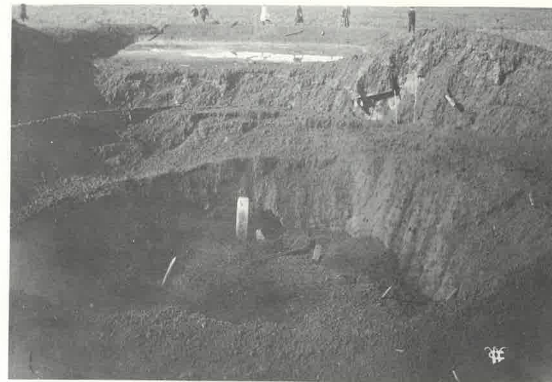
Alexander No. 1 Santa Fe Springs in 1922, showing crater after blowout that destroyed and buried drilling rig. Picture courtesy Richard Hathaway and Chas. A. Waer.
